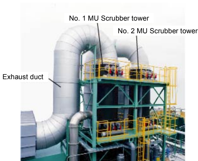
Figure 6 Wet deodorization system
