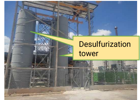
Photo-1 Full view of the site
