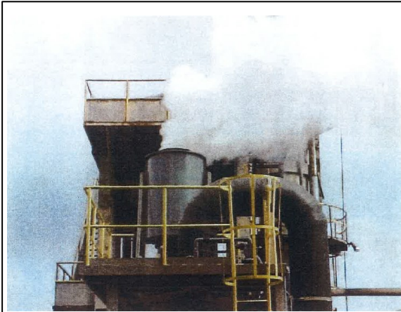
Photo 5 Prior to installation of MU Scrubber
