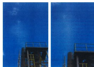
After deploying MU Scrubber
